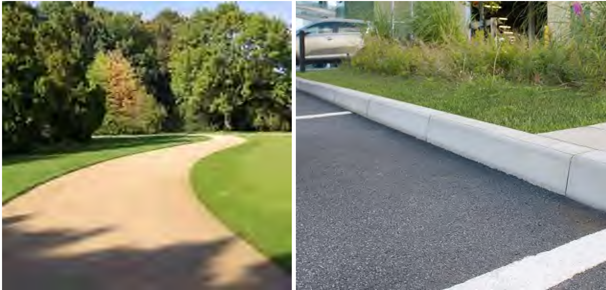
(Above) Example of hoggin path and typical concrete kerb
