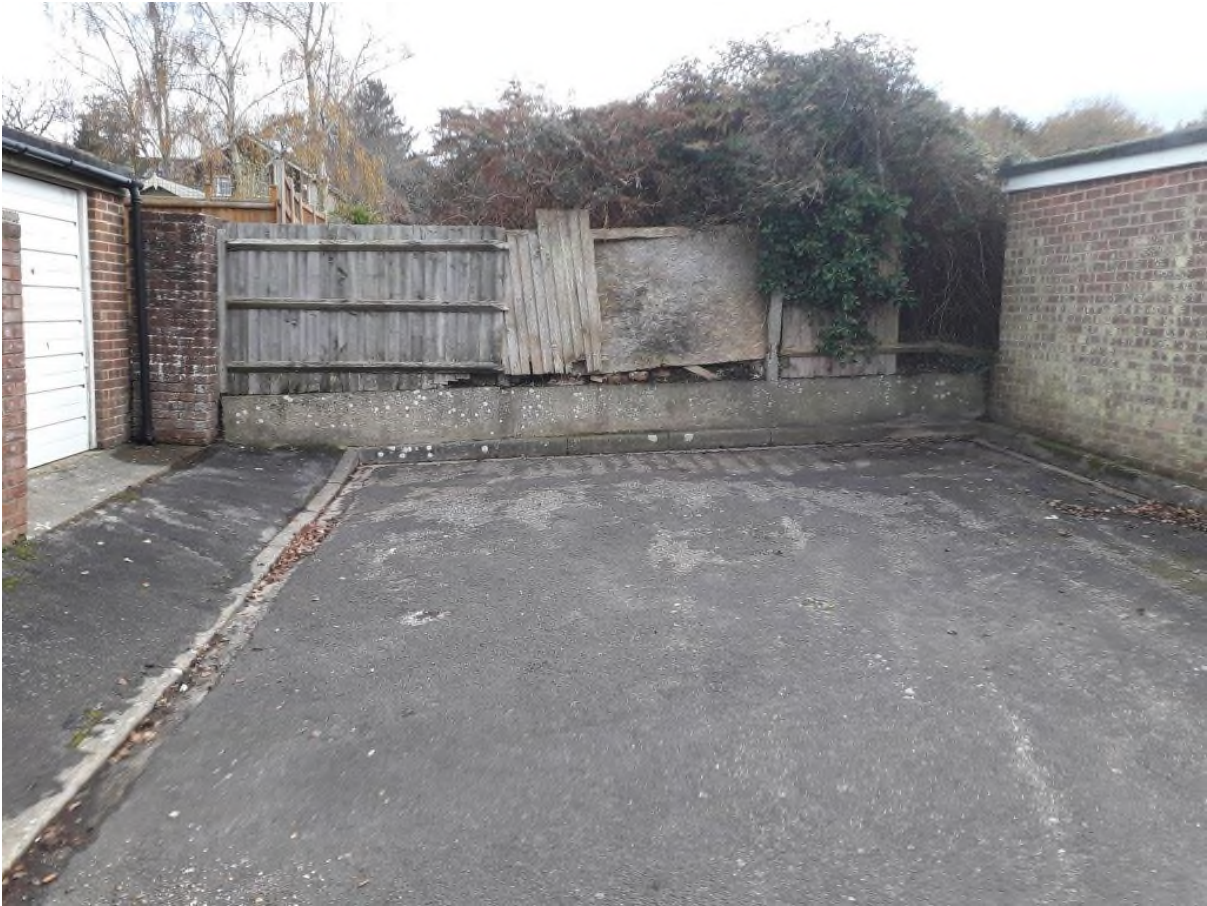
Figure 1 – Fence at rear of Frobisher Close
